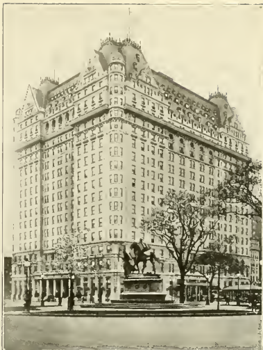
THE PLAZA HOTEL —Located on Fifth Avenue and 58th Street, facing Central Park and the Plaza. It is a model of elegance and beauty, 19 stories high and cost $12,500,000. It contains a beautiful Ball room accommodating 500 people.
